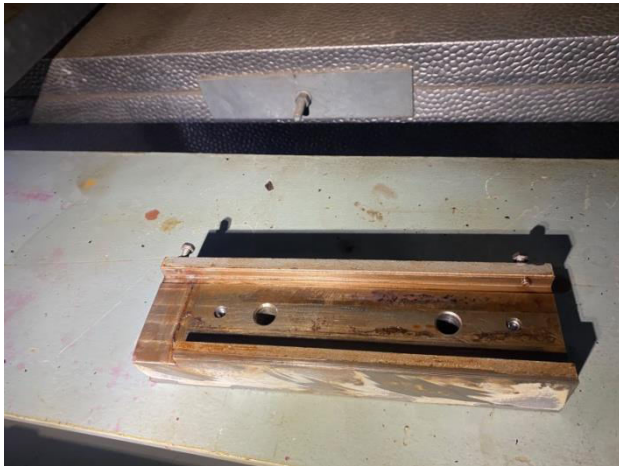
Rail section removed to enable bearing replacement.
