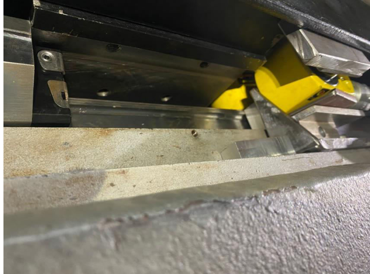
Z and Y direction press plates in place with the second bearing replacement.
