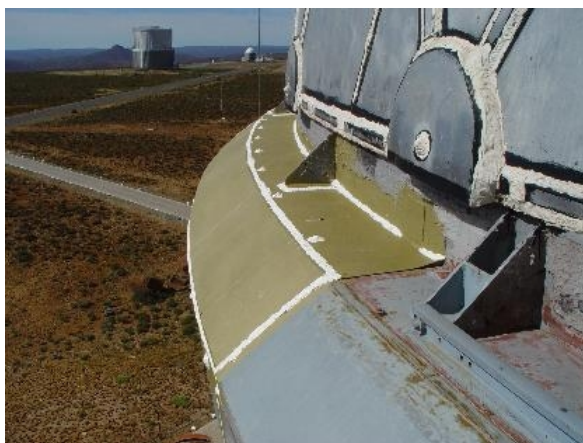
Re-sealing and painting work in progress on the dome.
