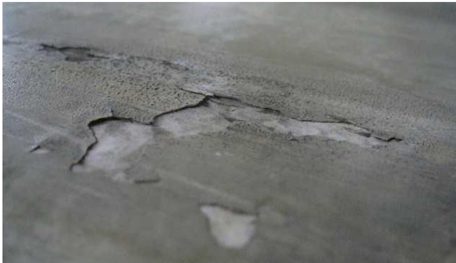
Delamination of the pier surface, which has now been repaired.
